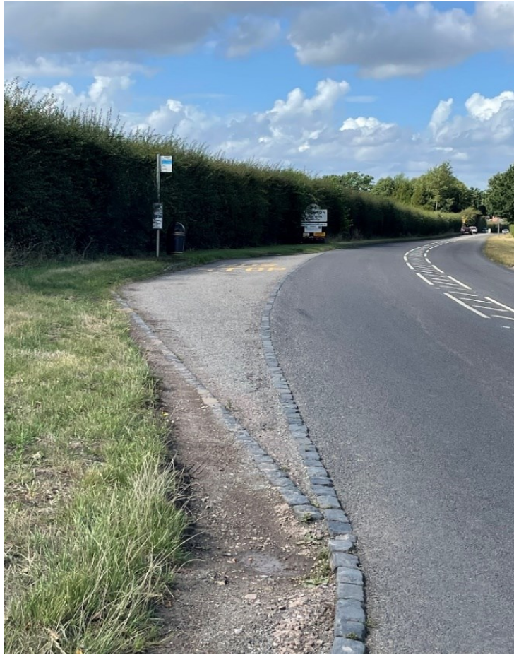
Figure 8: Bus Layby, Westbound - Haughton, Staffordshire
