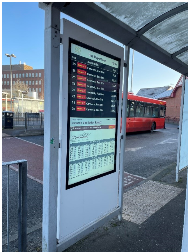
Figure 14: Integrated RTPI Screen - Stand 2, Cannock Bus Station
