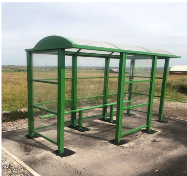
Figure 7: 3-Bay, Enclosed Bus Shelter
