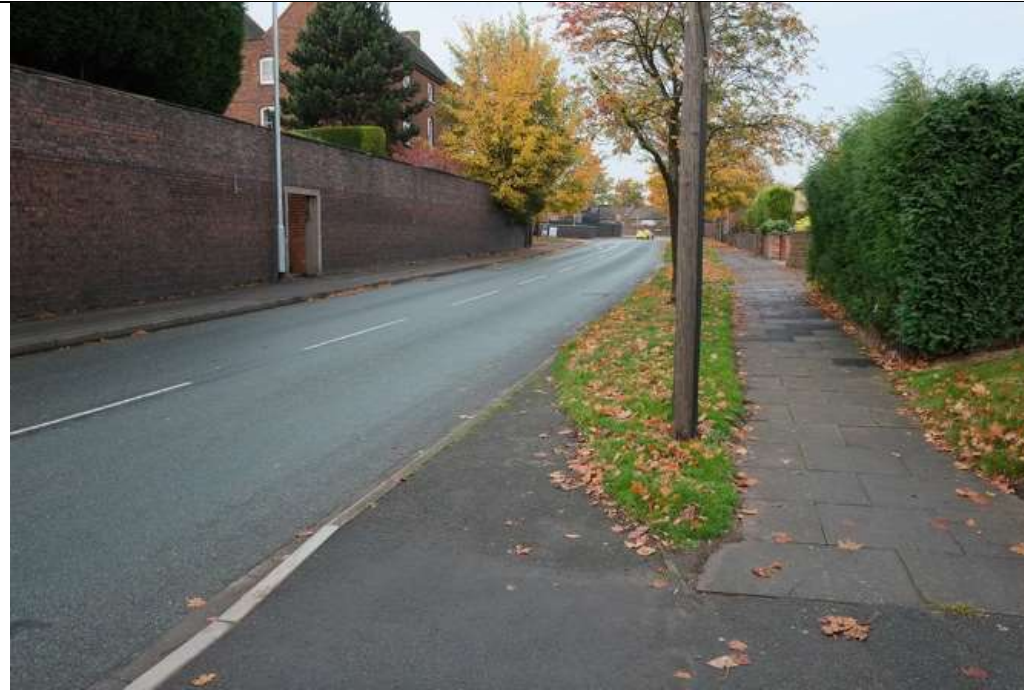
Hockley Road looking north at Tinker's Green Road
