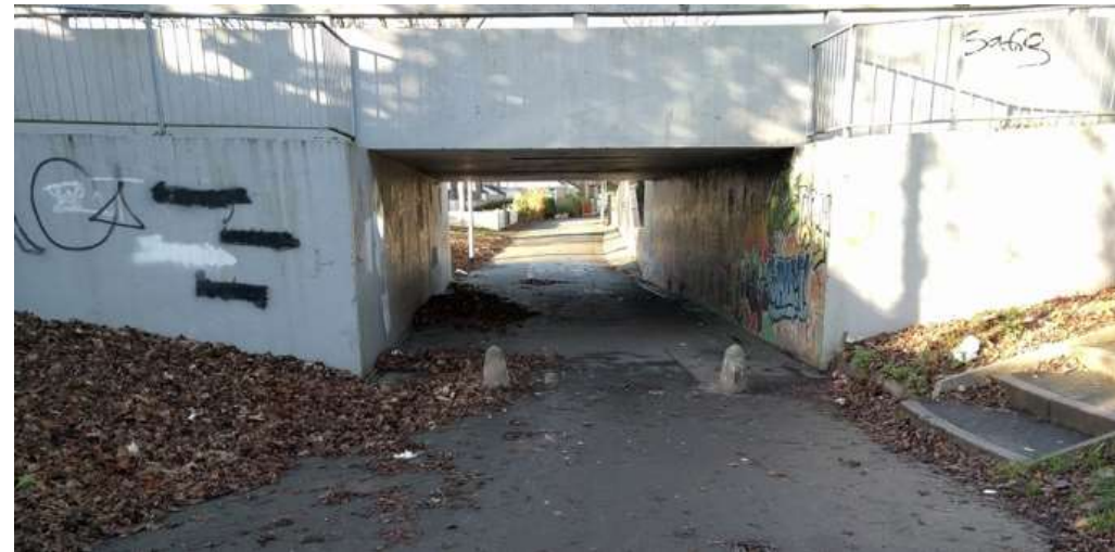
Underpass – Silverlink Road.
