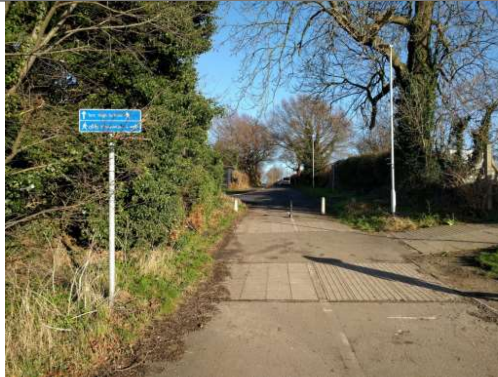
Cycleway over A5 to South Staffordshire College
