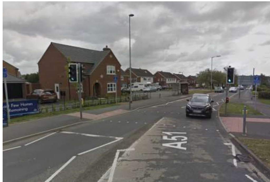
New toucan crossing at Peeler's Way
