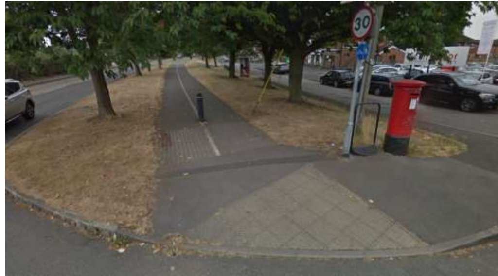
Segregated cycle route at Sutton Avenue
