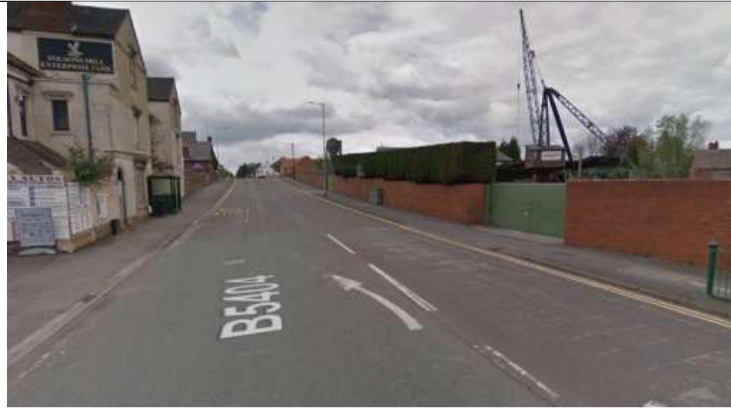
Lichfield Street looking west over canal bridge
