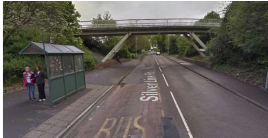
Cycle route bridge crossing Silver Link Way
