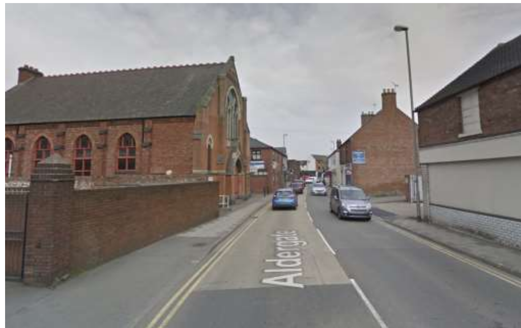
Aldergate looking north
