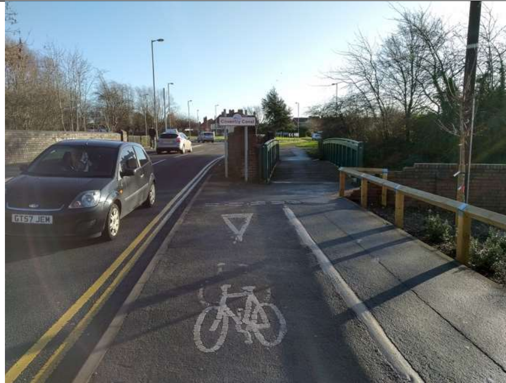
Missing gap in cycle route over the Coventry Canal
