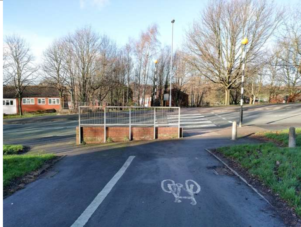
Crossing of Fossdale Road.
