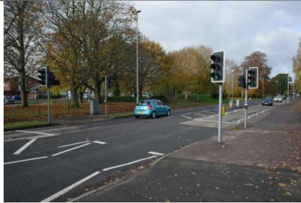
Pedestrian crossing on Cannock Road adjacent to Bridle Road
