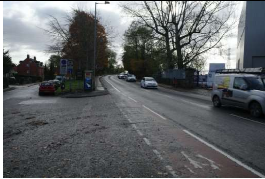
On-highway mandatory cycle lanes over railway bridge
