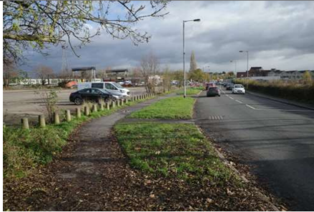
Doxey Road looking towards railway bridge
