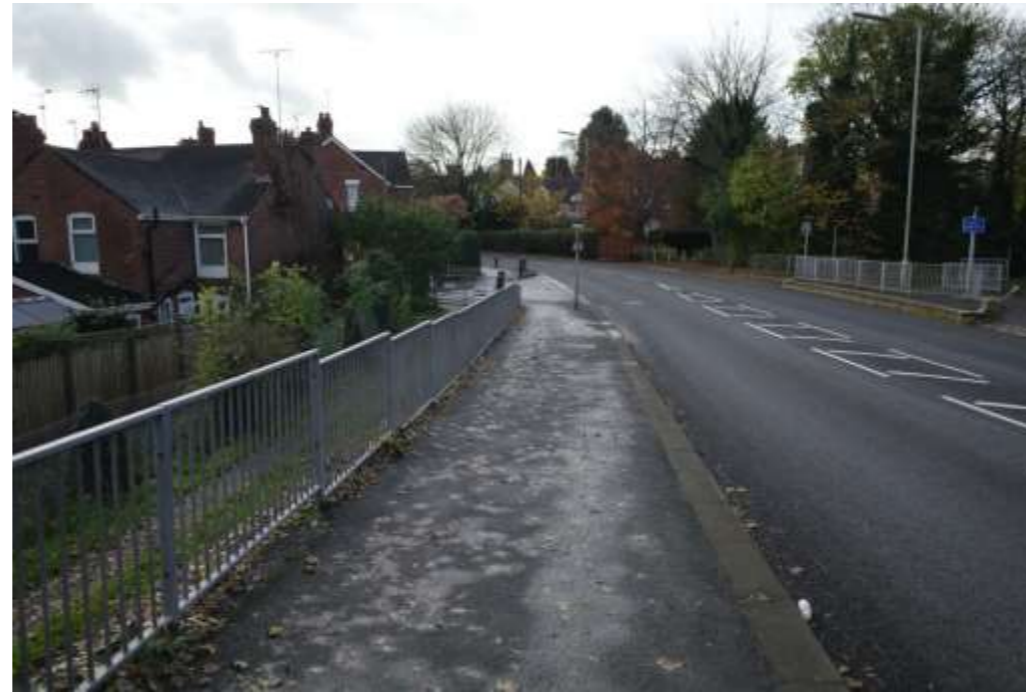
Wolverhampton Road towards Park Crescent
