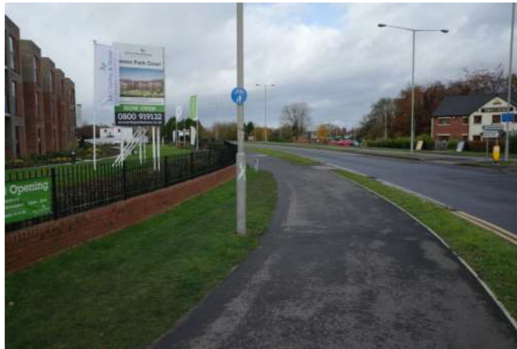
New shared use footway/ cycleway on Kingsway
