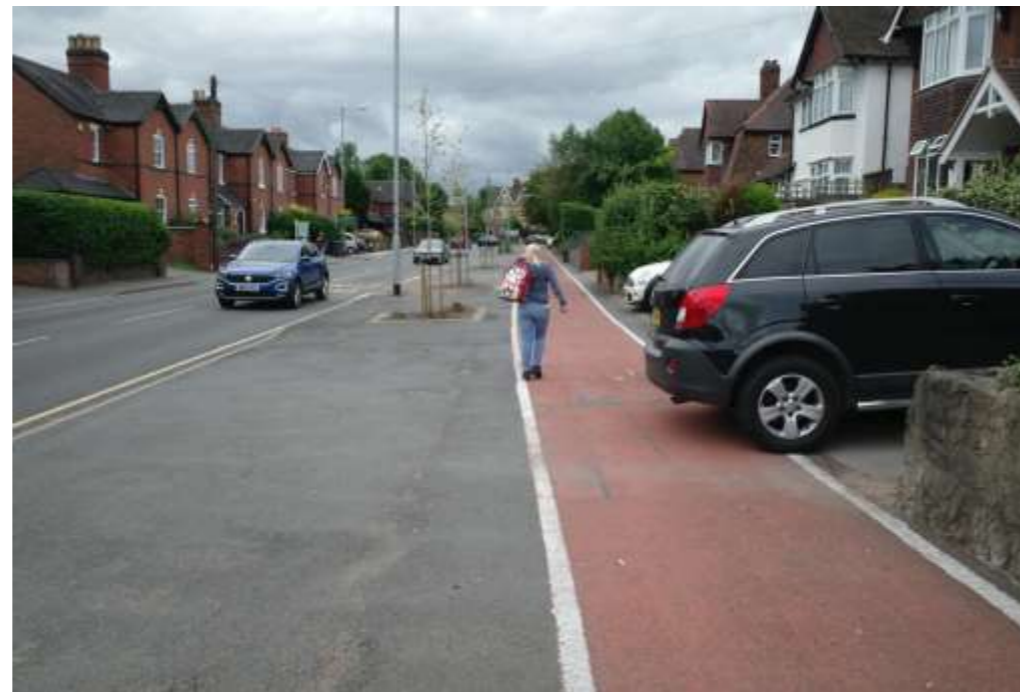
Existing cycle provision on Birmingham Road.
