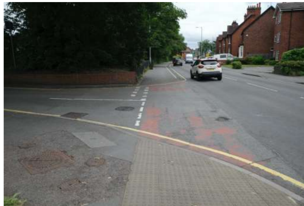
Existing cycle provision on Birmingham Road.
