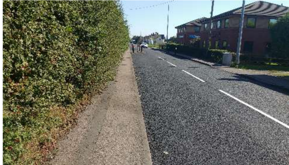
Cannock Road recent resurfacing and lining.
