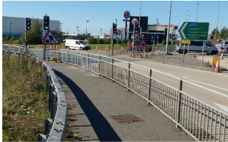
A5 Dumbell roundabout looking towards the Gateway Retail Park.
