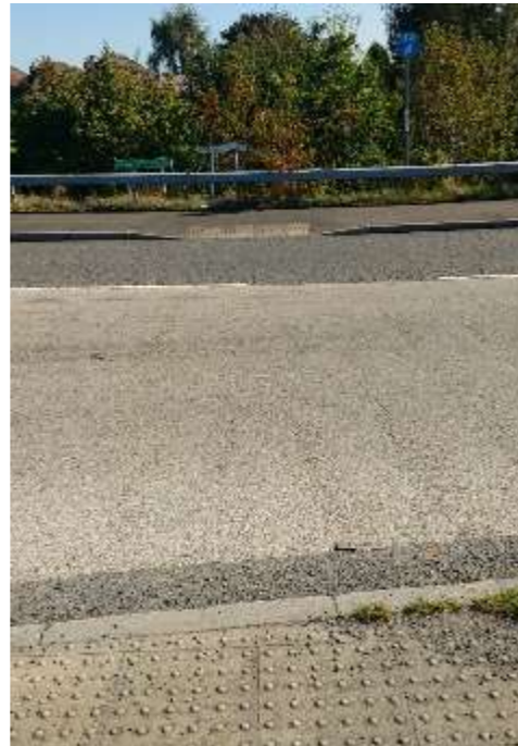
Walsall Road crossing point.
