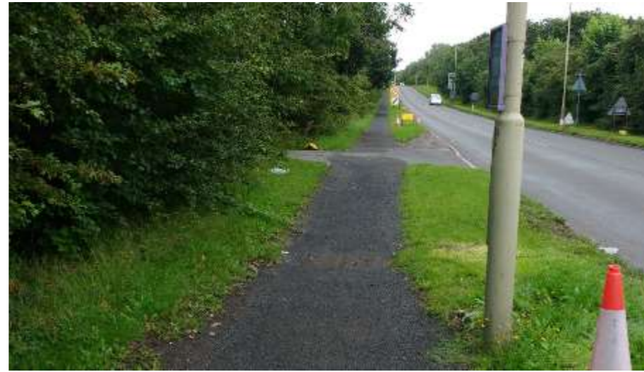
Lichfield Road, East of the A460 roundabout.
