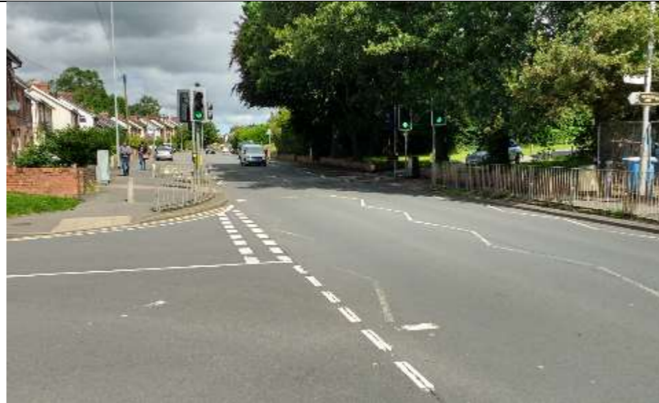
Stafford Road, Cardinal Way junction.
