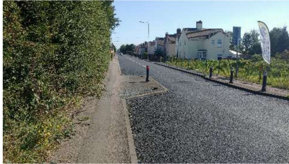
Cannock Road Traffic Calming.
