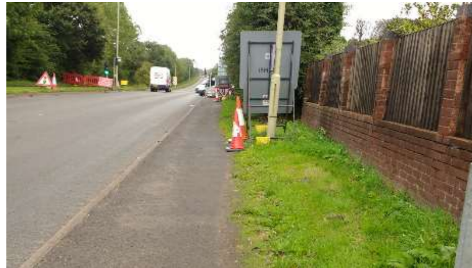
Lichfield Road, East of the A460 roundabout.
