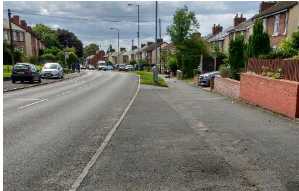
Stafford Road footway looking south.
