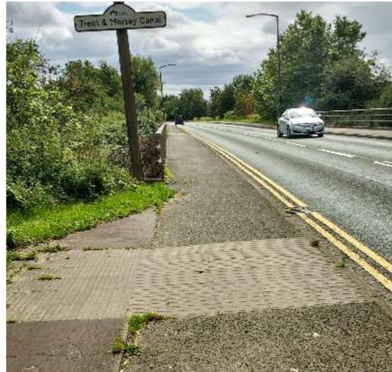
Princess Way, Canal Bridge narrowing.
