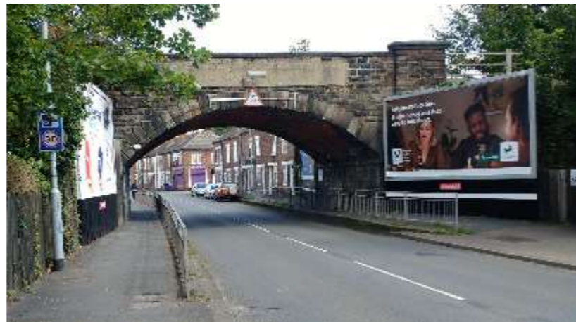
Branston Road Railway Bridge.
