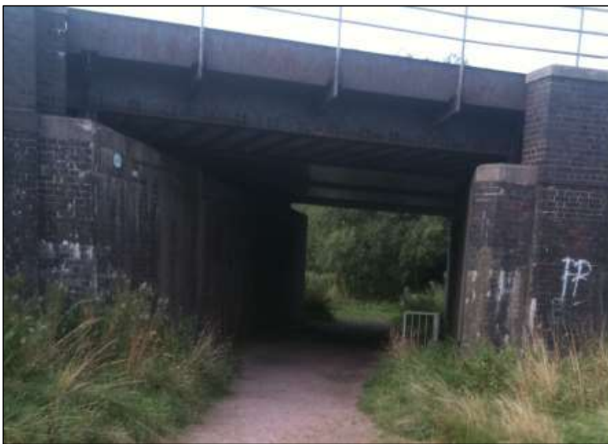
Figure 16: Underbridge UB78 beneath the West Coast Mainline
