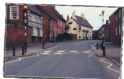
Pedestrian crossing combined with speed controlling devices - Abbots Bromley
