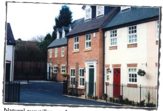
Natural surveillance of an entrance
