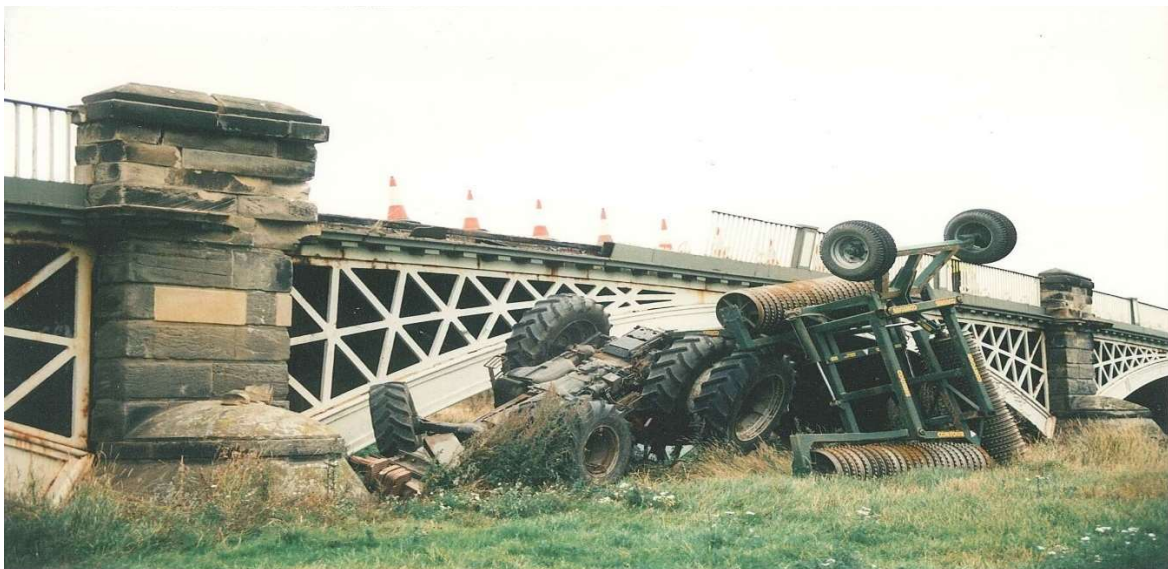
Figure 10 – Chetwynd Bridge Vehicle Strike
