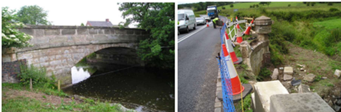
Figure 13 – Burndhurst Bridge, Loxley
