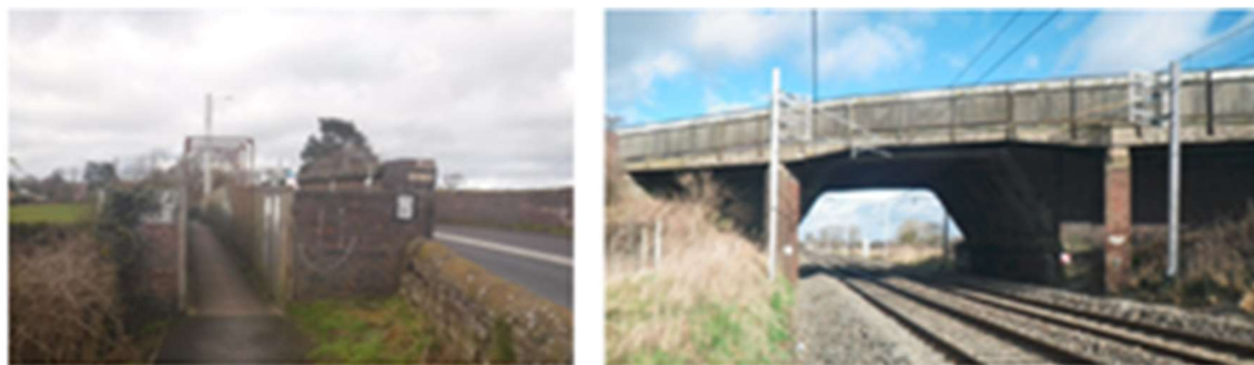
Figure 6 – Moss Pit Footbridge Images
