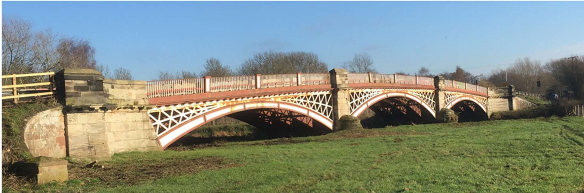
Figure 9 – Chetwynd Bridge, Alrewas
