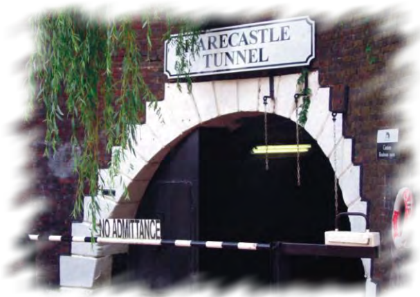
Harecastle Tunnel entrance
