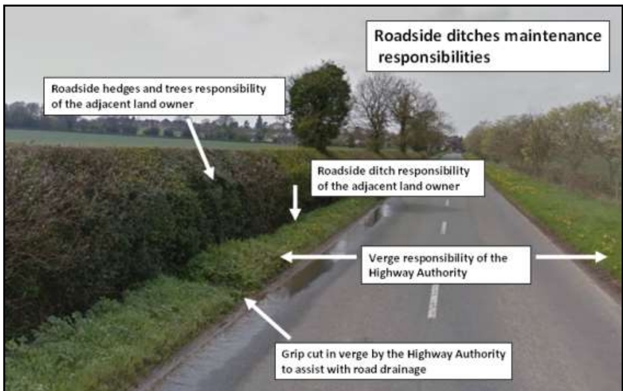
Figure 5-1: Responsibilities for Roadside Ditches and Watercourses
