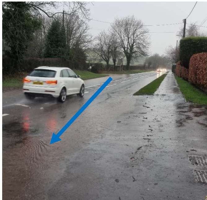
Figure 25: Surface water beginning to accumulate at junction of Aspley Lane and A519 and starting to flow in a southerly direction (blue arrow) down the A519 (Photo looking in a northerly direction) (Photo provided by resident)
