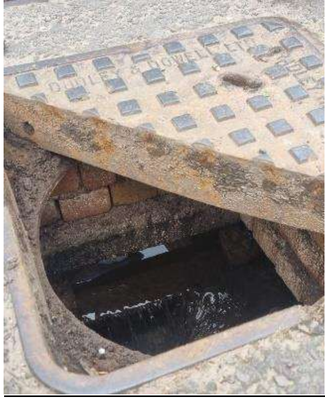
Figure 12: Weir in manhole at top of Villa Farm Lane
