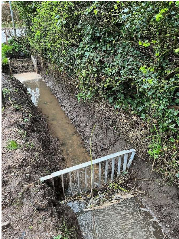
Figure 34: Two-stage trash screen installed along roadside ditch pipe inlet at Aspley Lane/A519 in February 2024
