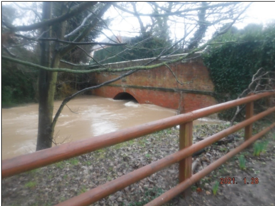
Figure 15: High river levels at Town Hill Bridge during Storm Christoph, January 2021
