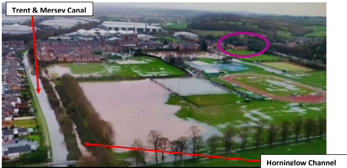
Figure 9: Flooding to the Leisure complex fields to the rear of Price Court (pink circle). Photo is looking in a southerly direction towards Price Court. (Source: Photograph provided to SSC LLFA by representatives from Shobnall Leisure Centre. The exact date and time of the photograph is unknown).
