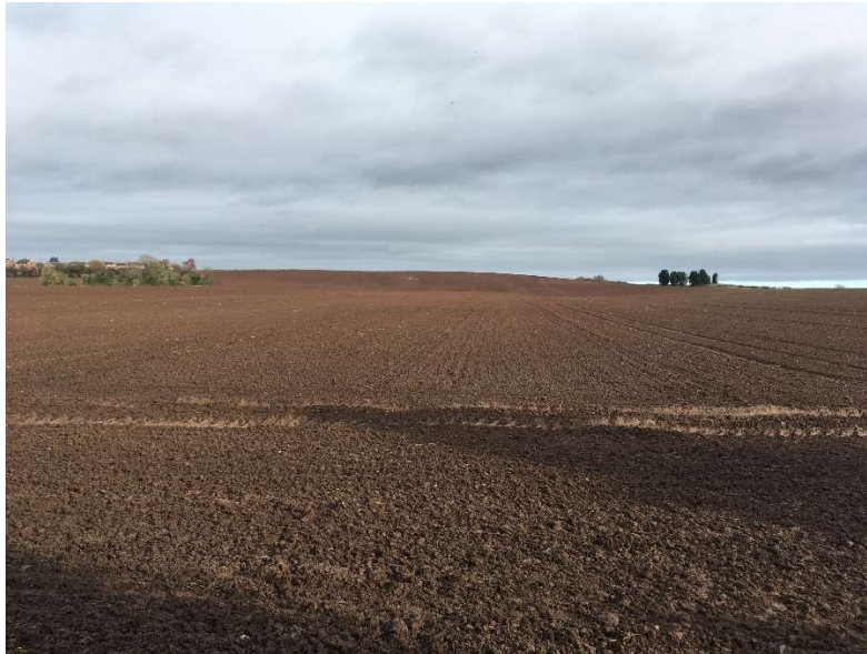
Figure 14: Looking in a northerly direction across the field from Culvert A (Photograph taken in November 2020)
