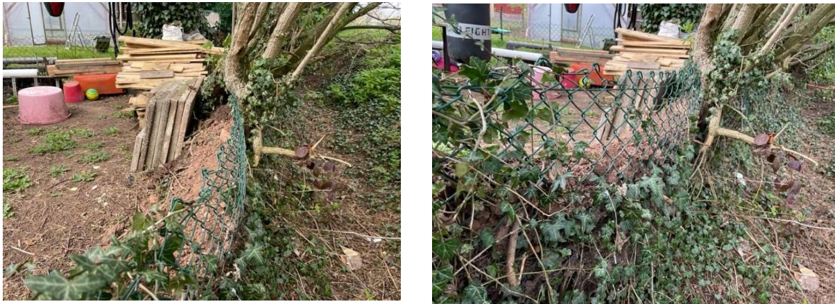
Figure 20: Photographs demonstrating the informal bund between drainage ditch and gardens of properties along Mead Crescent
