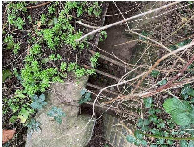
Figure 17: Trash screen situated above culvert outlet pipe A
