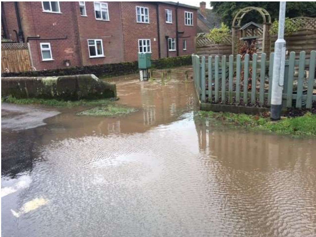
Flooding at Church Lane road bridge, Marchington
