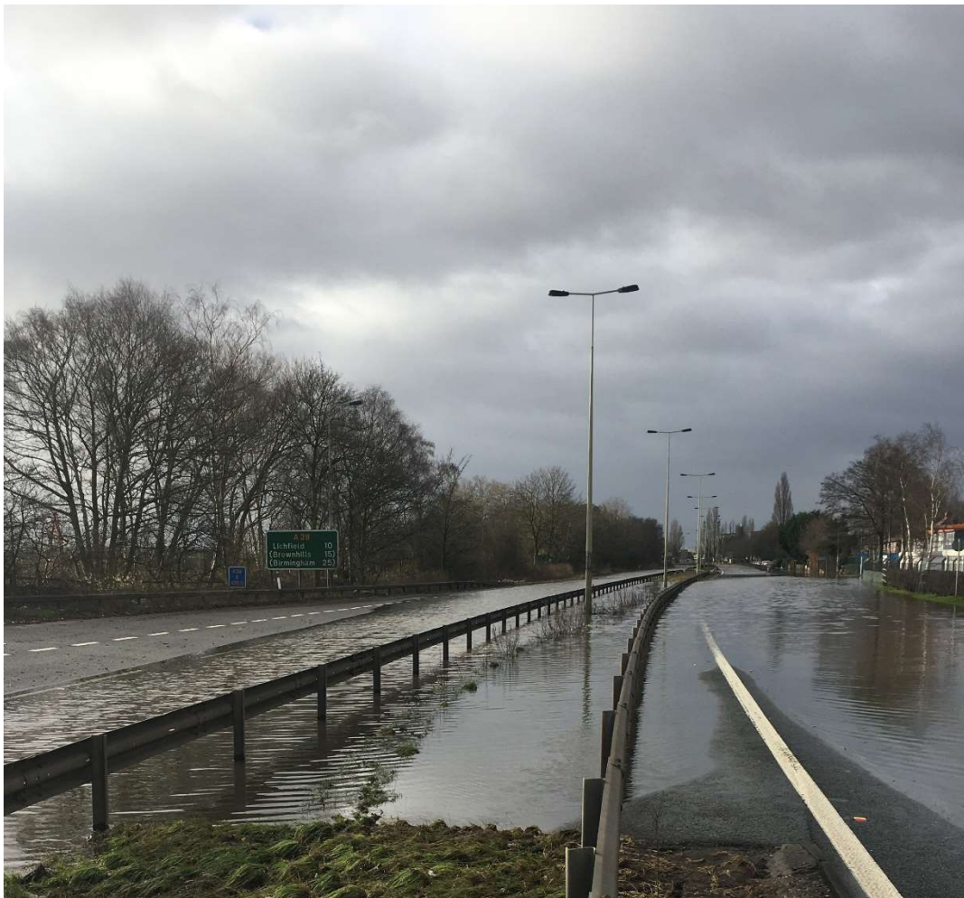
Figure 1: Flooding on the Lichfield Road section of the A38 (image source and rights belong to the Environment Agency)
