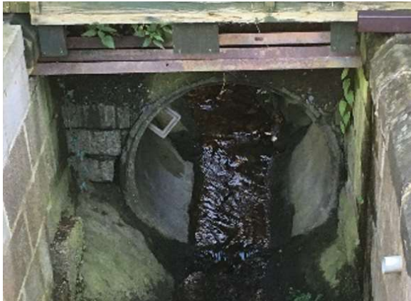
Figure 15 - Culvert 2: Approximately 1000mm diameter
