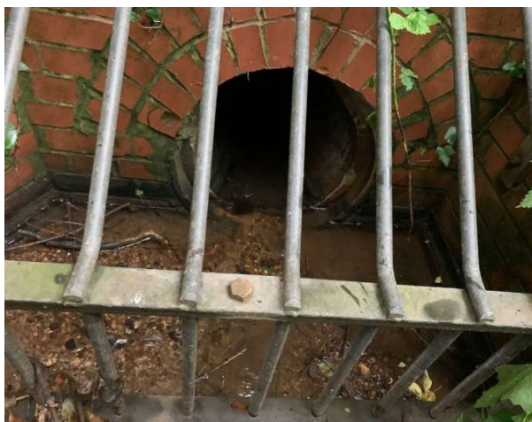
Figure 14 – Culvert 1: 450mm pipe and trash screen at eastern footpath crossing
