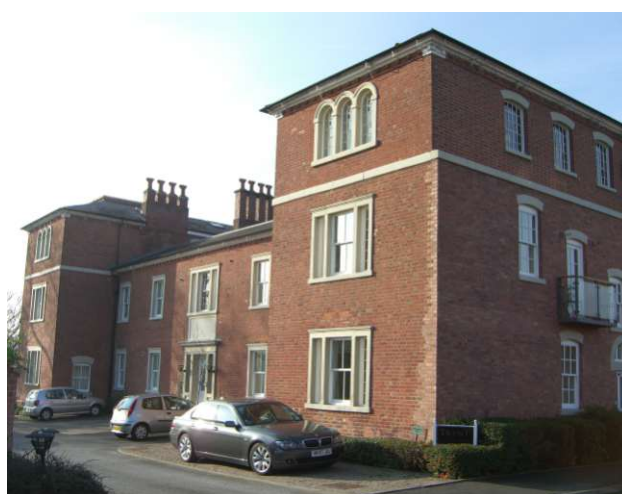
Plate 5: The former Workhouse
