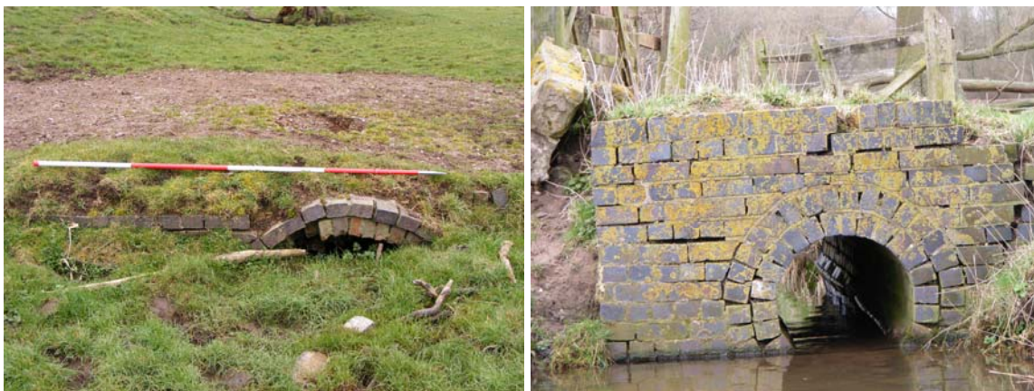
Figure 50- 19th century culvert and bridge features, Cresswell Farm
