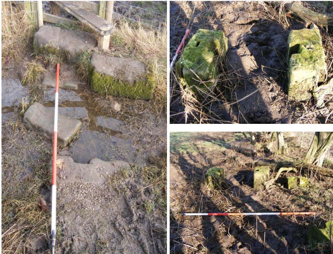
Figure 60- Preserved sluice hatch settings, Willows Farm
