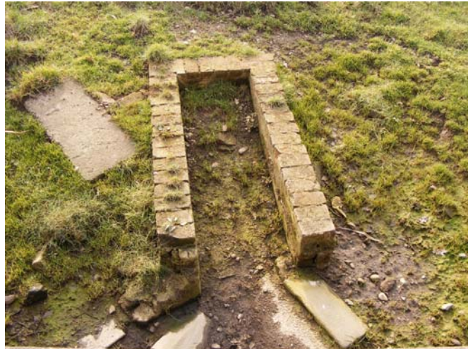
Figure 21-Unknown brick structure in proximity to historic sluice location-Great Haywood
