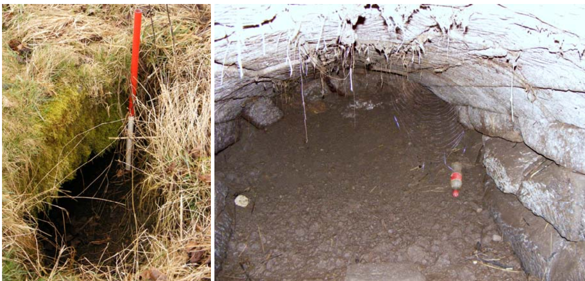
Figure 62- Preserved bridge, Willows Farm, external (left) and internal views (right)
