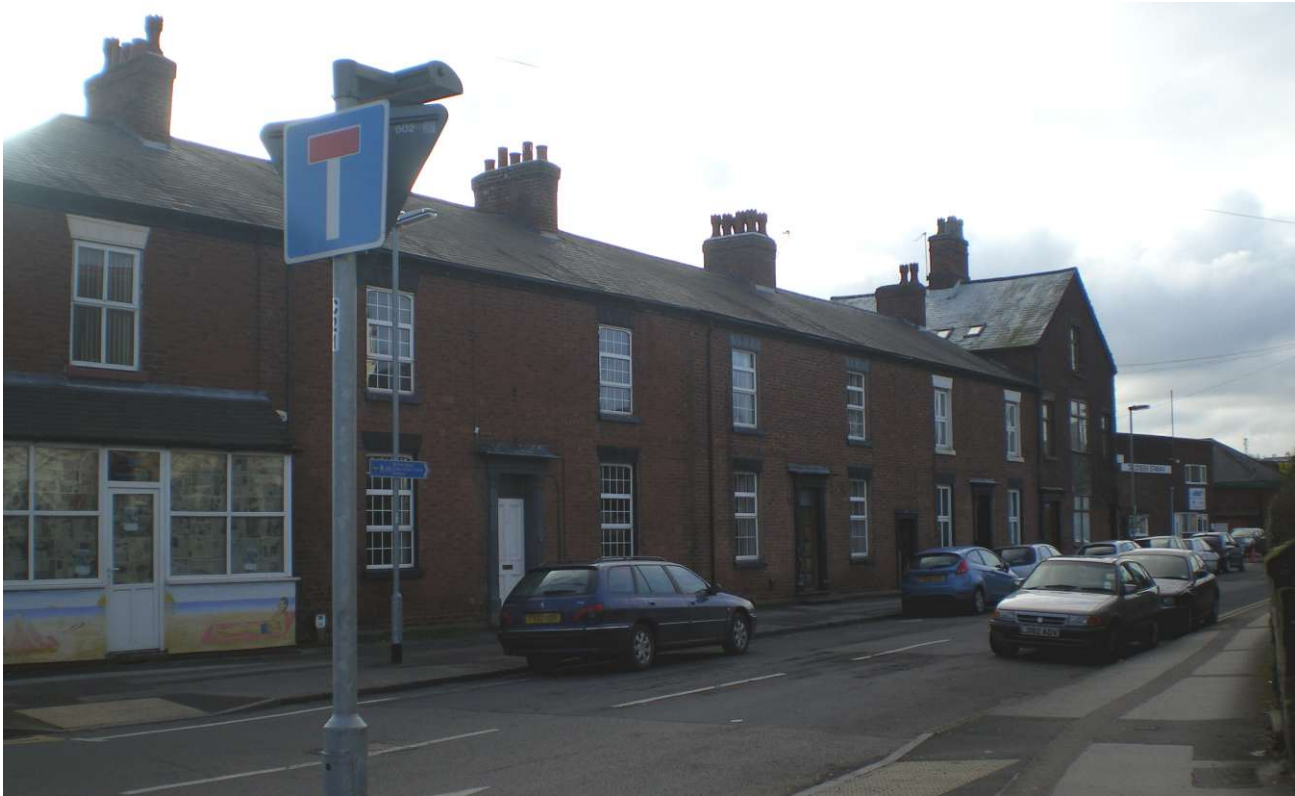
Plate 12: 19th century properties in Market Street
