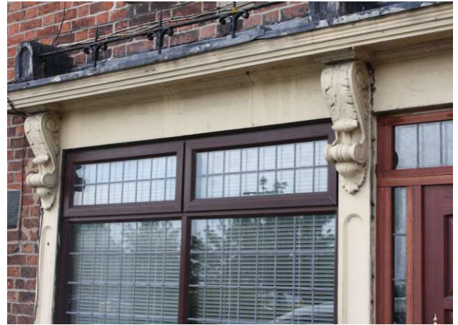
Plate 7: Possible 19th century shop front, High Street. © Staffordshire County Council
