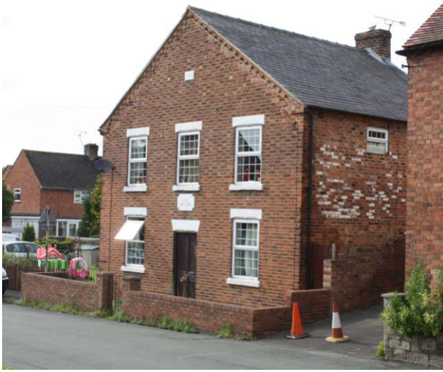
Plate 9: Former Baptist Chapel on Church Lane with date stone of 1889. © Staffordshire County Council
