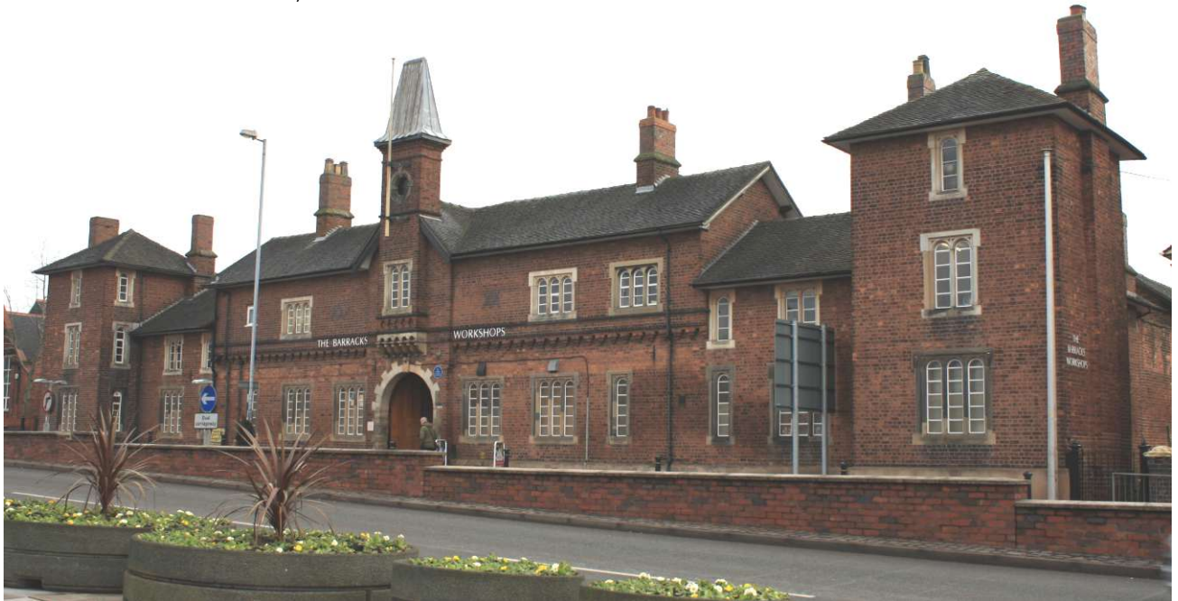
Plate 15: The former Barracks, Barracks Road
