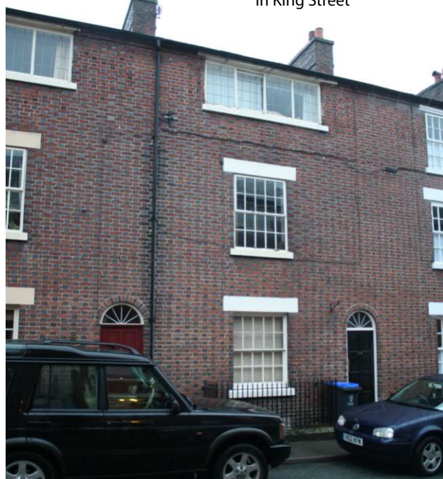
Plate 9: Weavers' Houses in King Street
