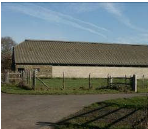
Figures 32 and 33 Purpose-built covered yard buildings
