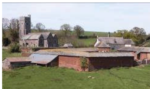
Figure 9 A Regular Courtyard farmstead in Devon with linhays (two storey open-fronted shelter sheds with haylofts above) which has no openings in the external elevations.
