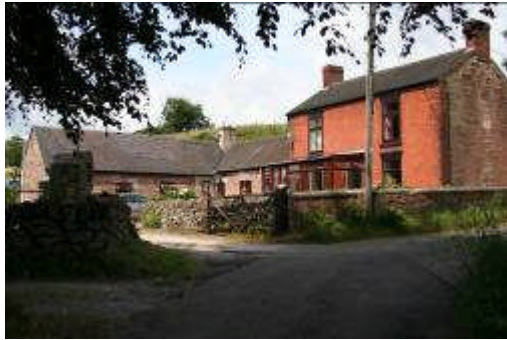
Figure 46 Small L-plan range with later farm buildings attached to the house (which has been re-faced with brick).
