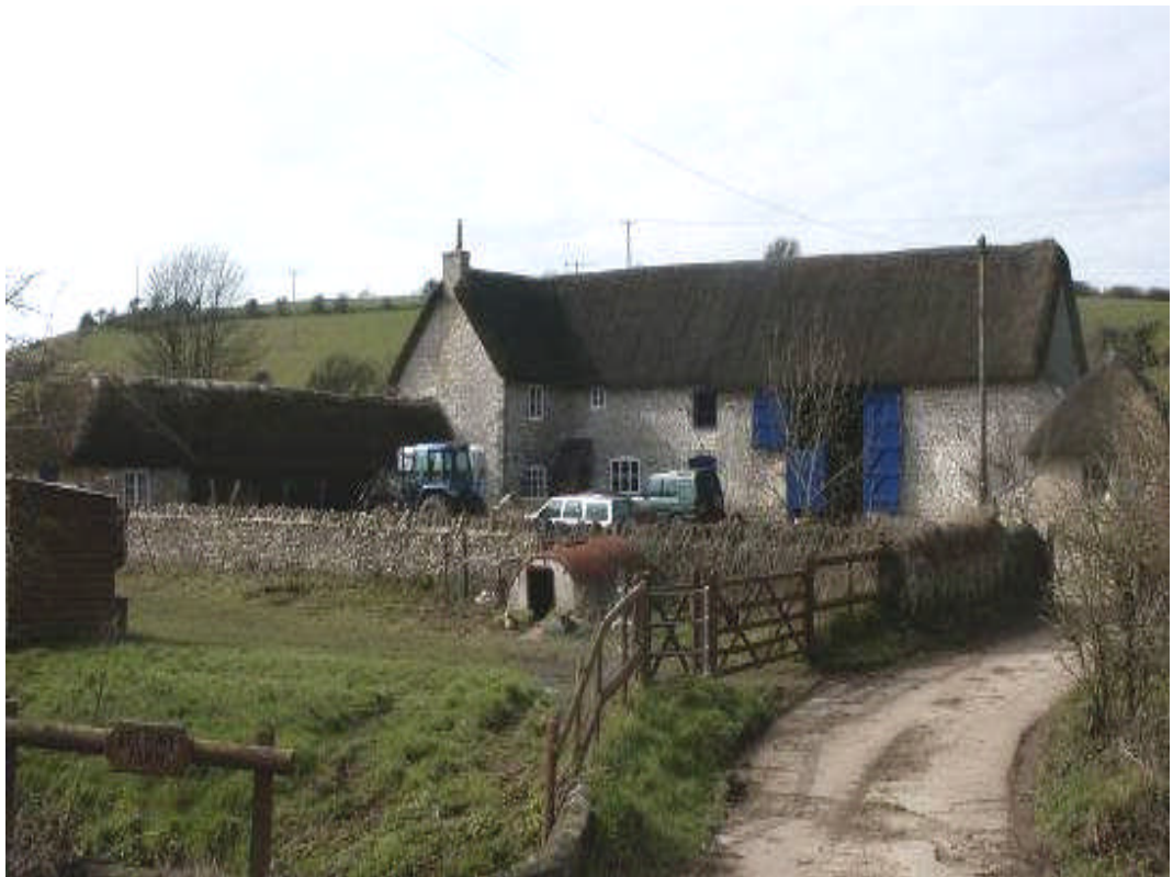
Figure 47 An L-plan range with house, stable and barn built in a single phase and a single storey cartshed attached to the house.
