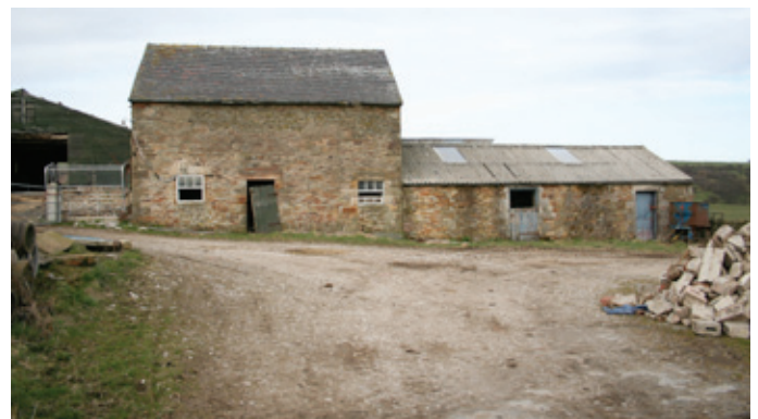
An early to mid 19th century storeyed cow house with later single storey extension. Photo © English Heritage
