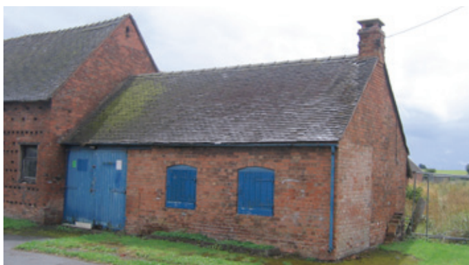
Single-storey smithy fronting onto village street, but attached to a range of farm buildings. Photo © Jeremy Lake
