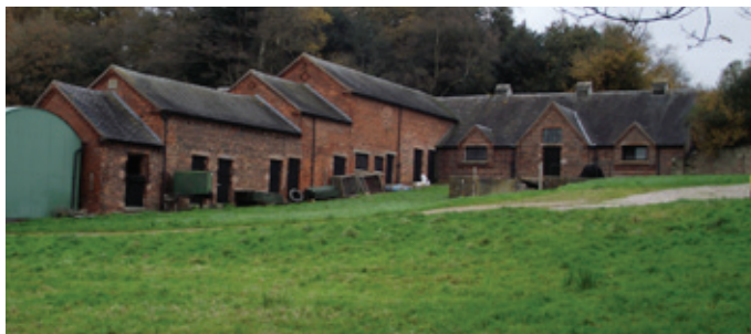
An L-shaped range of cattle housing, all built in different phases between the mid 19th century and (right) the 1920s-30s. Photo © Staffordshire County Council
