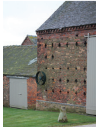
Occasionally evidence for the use of mechanisation for threshing and processing feed can be found in the form of external fly wheels and internal gearing power which were powered by portable steam engines. Photo © Bob Edwards
