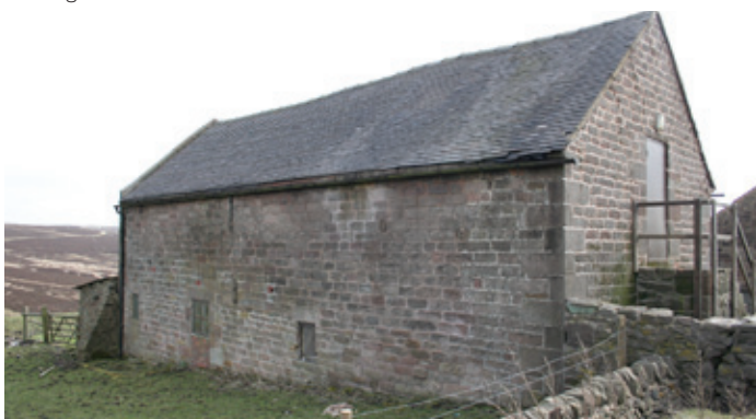
Steps to an upper floor granary and wool loft in the gable end of a combination barn. Photo © English Heritage
