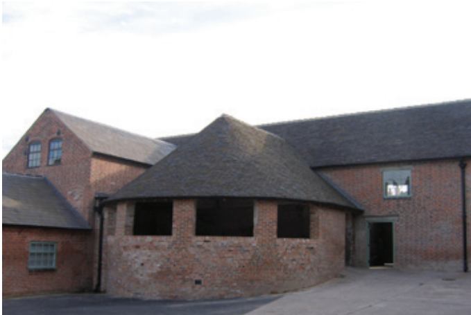
A wheelhouse with a conical roof projecting from a combination barn. Such survivals, which housed horse-powered machinery for threshing grain and processing fodder, are very rare. They were initially built on the largest farms, usually the home farms to estates. Photo © Jeremy Lake
