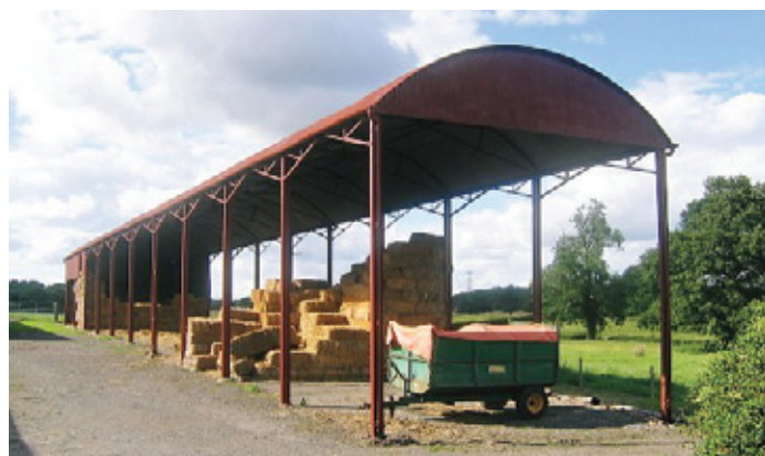
By the late 19th century mass-produced buildings were becoming available, the Dutch barn being the most commonly seen prefabricated building of the period. Photo © English Heritage
