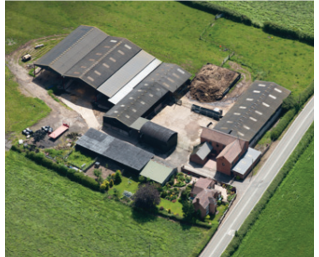
A small roadside farm, built to a regular courtyard L-shaped plan, which is located in an isolated position in western Staffordshire. This red brick farmstead dates to the 19th century and, with its cattle housing and hay lofts, is typical of small dairy holdings established during this period in this part of Staffordshire. Photo © English Heritage NMR 27999/007.
