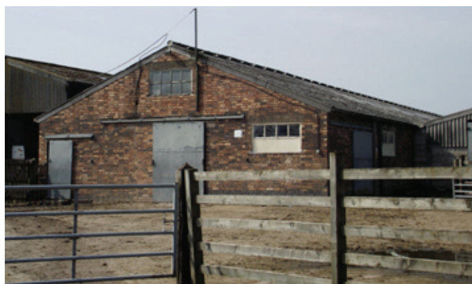
An inter-war dairy built from machine brick, these were commonly provided with metal truss roofs. Photo © Staffordshire County Council
