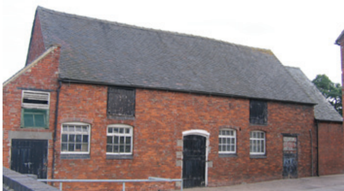
Many cow houses were converted from earlier barns and other buildings in the late 19th and early 20th centuries. The windows to this range have been inserted, and the metal frames conform to 1930s hygiene regulations. Photo © Jeremy Lake
