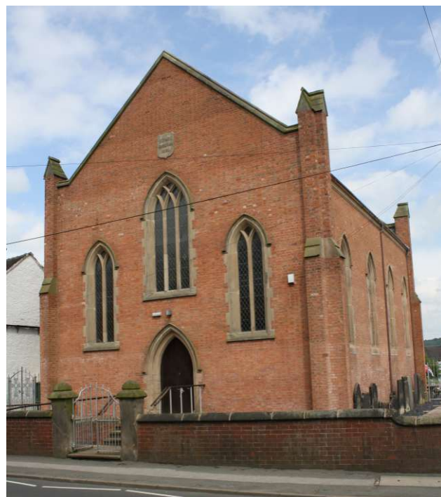
Plate 16: Congregational chapel, Tape Street
