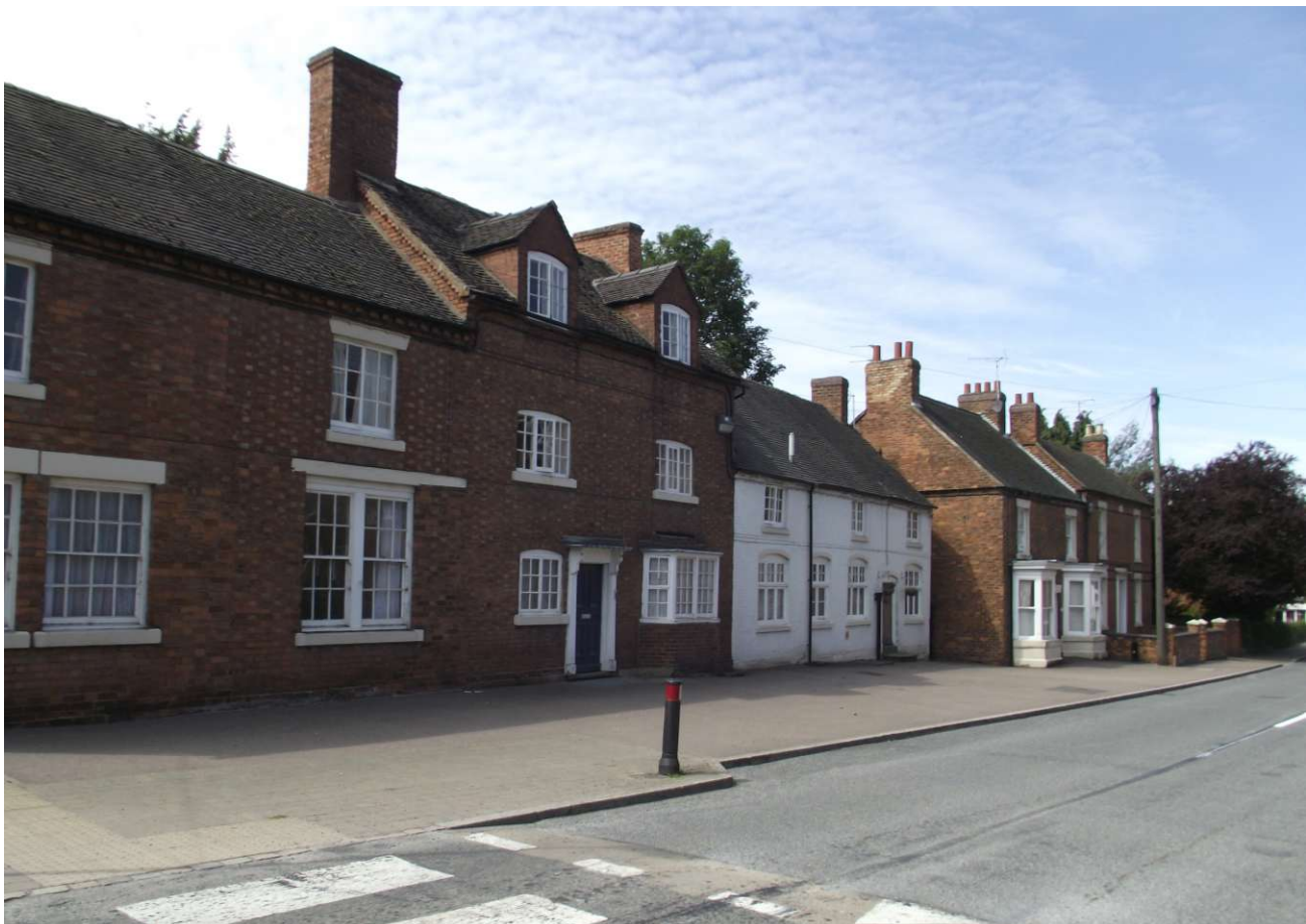
Plate 16: Southern side of High Street
