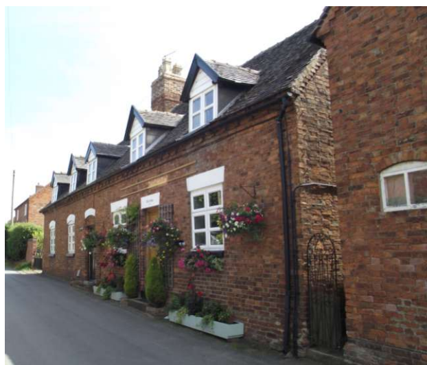
Plate 9: Oak Cottage and The Cottage; possibly the former Parish Workhouse
