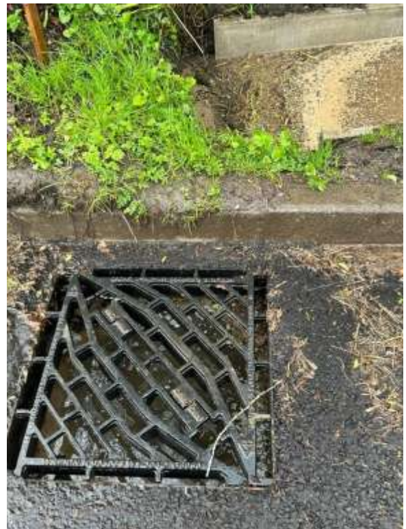
Figure 37: Gully adjacent to Aspley Lane ditch almost at capacity following rainfall April 2024
