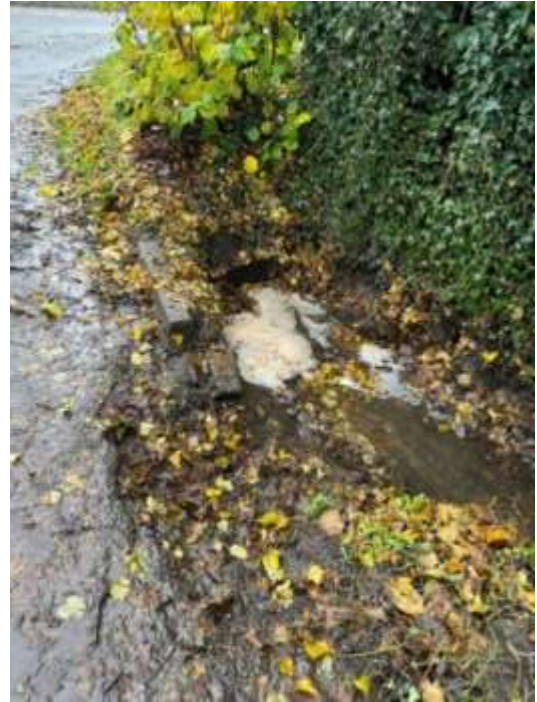
Figure 24: Blocked trash screen at Aspley Lane pipe inlet (Photo provided by resident)
