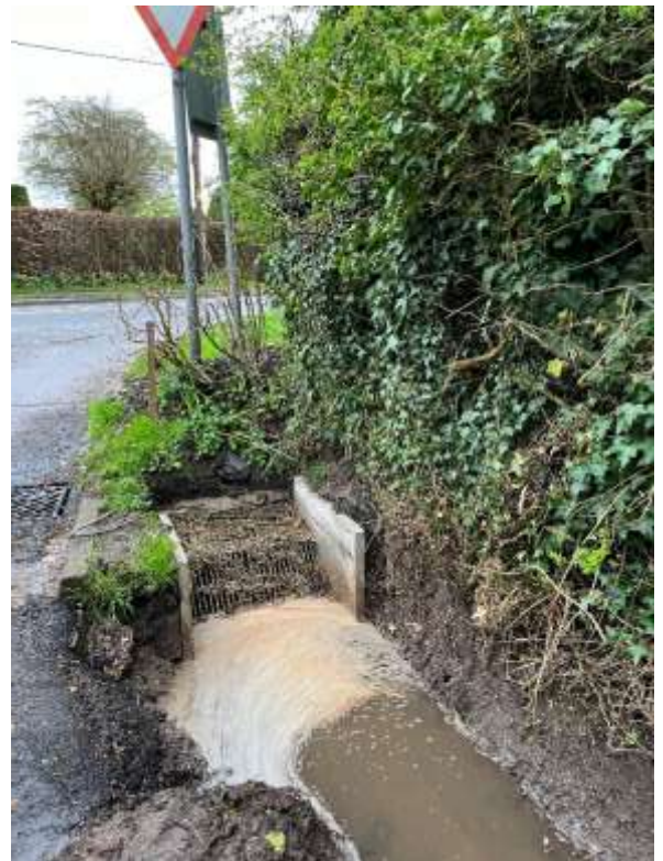
Figure 35: Aspley Lane inlet pipe and new trash screen following heavy rainfall February 2024.
