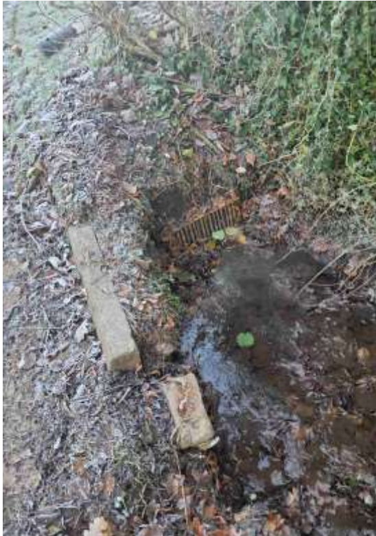
Figure 11: Trash screen on inlet to Aspley Lane pipe
