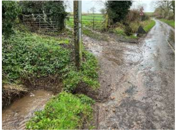
Figure 30: Surface water runoff from fields adjacent to Aspley Lane, observed on 22 nd February 2024
